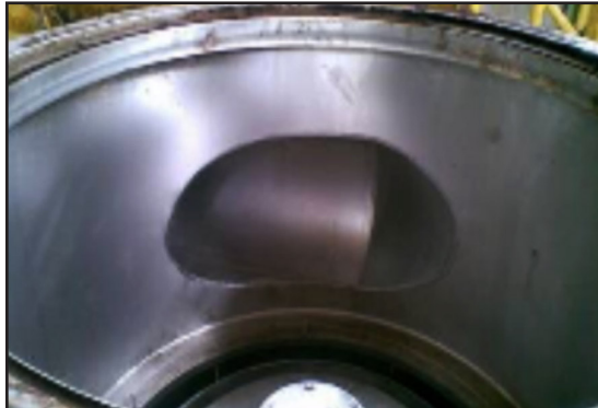
Screen housing after surface prep
