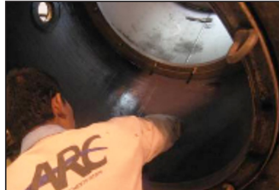
Application of ARC BX1*
